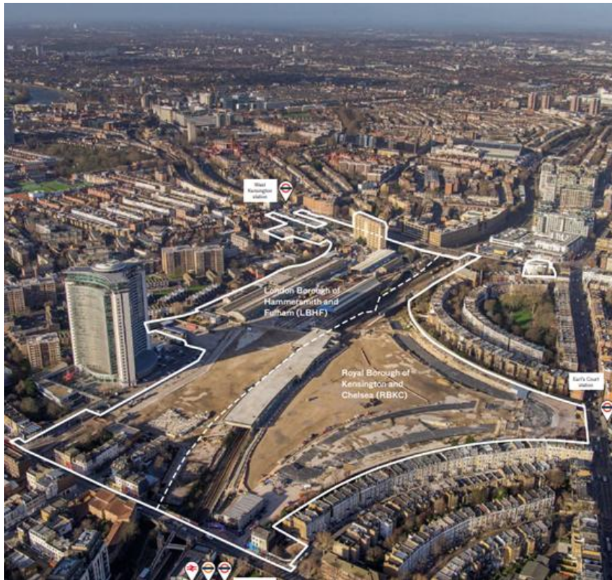
Figure 3: Aerial View of the Earls Court Development Site
