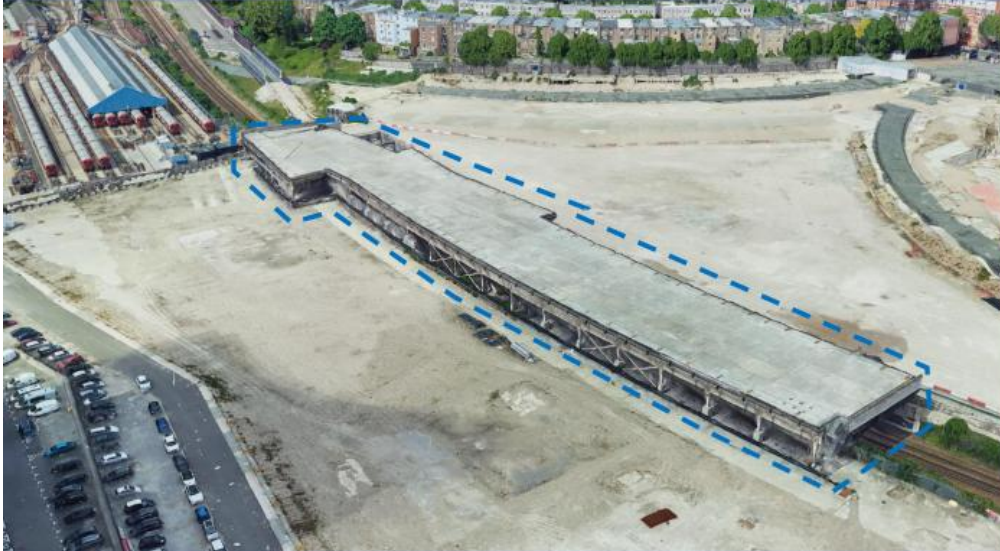
Figure 4: Existing retained deck on the site
